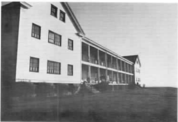
Our sleeping quarters, an historic barracks hall, remodeled into separate small rooms.
